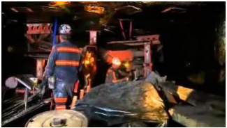
Supporting mine roof with roof bolts
